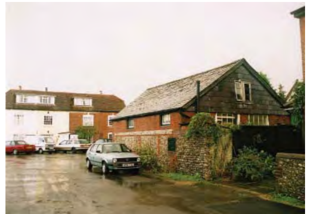
Non designated heritage asset outbuilding in Church Road
