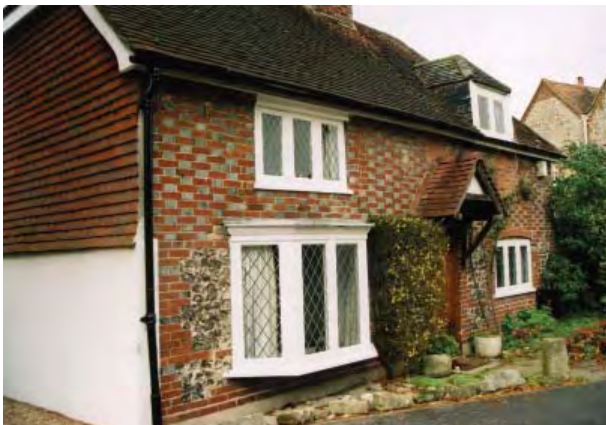
Mill Brook Cottage, Church Road
