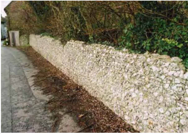
Stone wall in River Street
