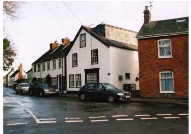
Over-sized “dormer” at No. 1a River Street
