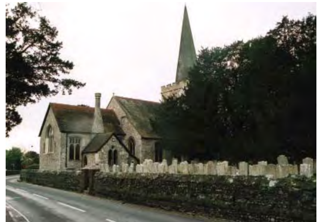
St John the Baptist's Church from Westbourne Road
