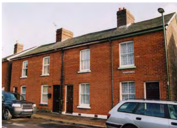
Non designated heritage assets in North Street
